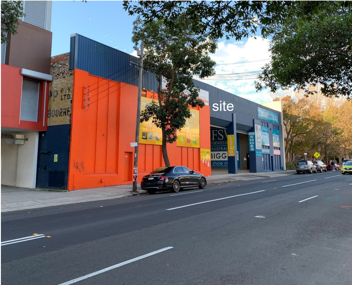
looking east along McEvoy Street
